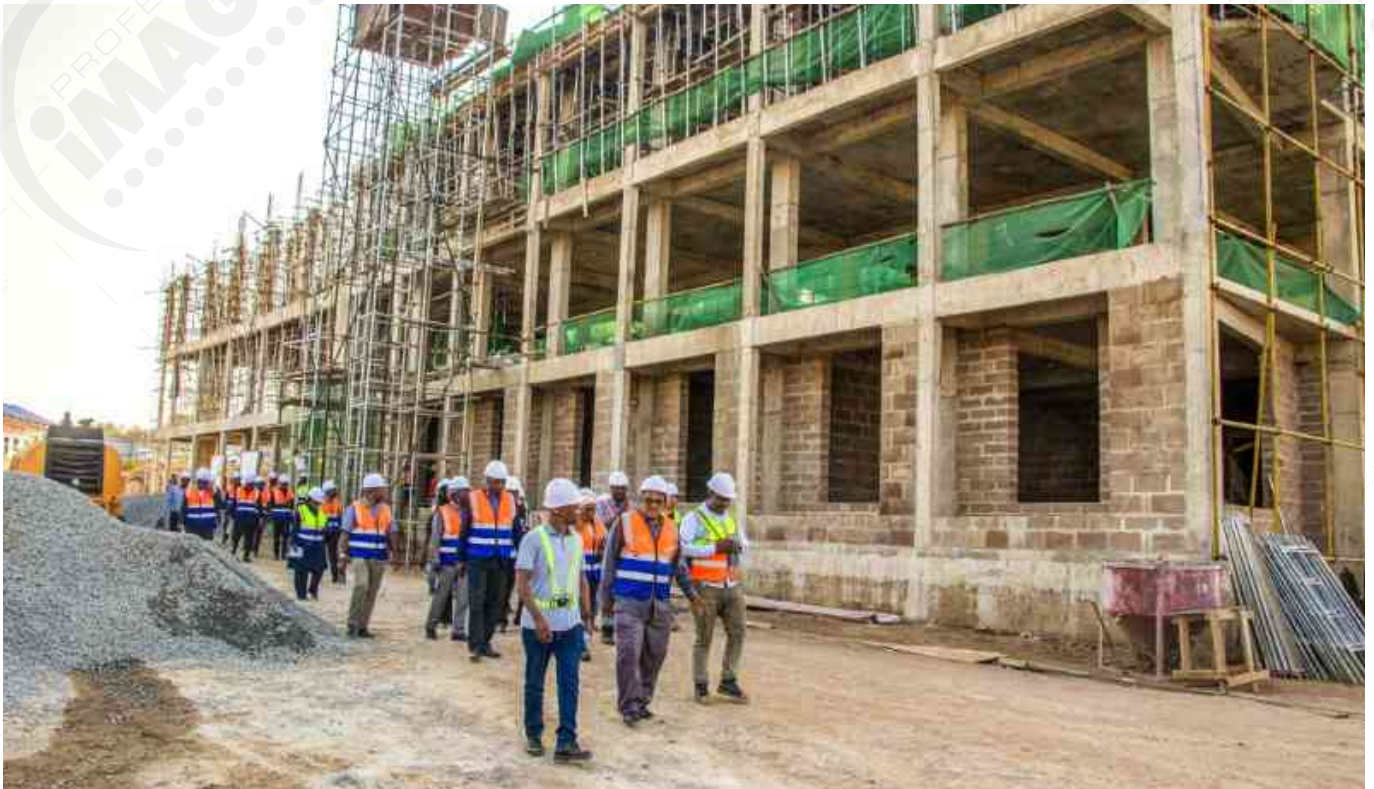
TBS Board Chairman Prof. Othman Chande Othman (centre) leads members of the TBS Board of Directors and service providers during a recent inspection of the Bureau's new laboratory and office complex under construction in Mwanza.
